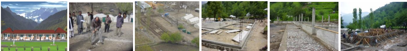
GHS – Bhunja Proposed Model, Ground Breaking and Construction Work in Progress
