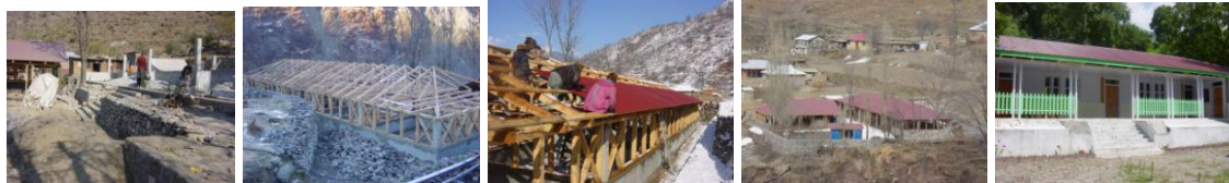
GGPS – Bhunja, Construction Work in Progress
